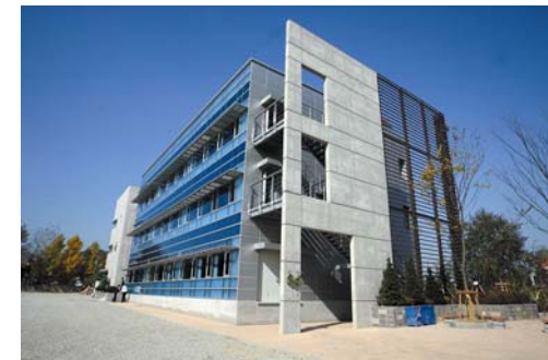
South Korea: Kolon R&D Institute of Technology Building
